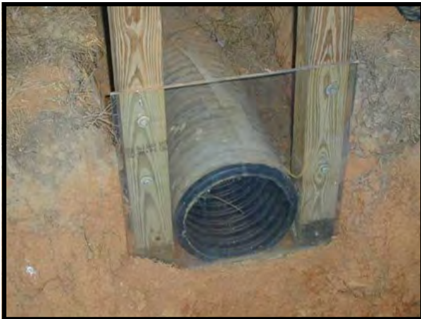
Filter wrapped 10" inch perforated corrugated pipe.
