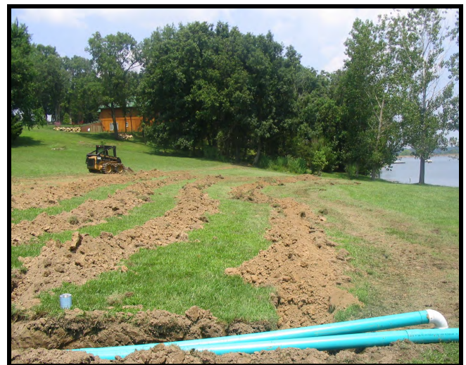
Dispersal trenches installed on contour.
