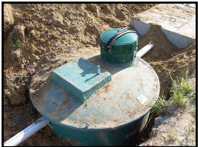
Installation of an aeration treatment unit.
