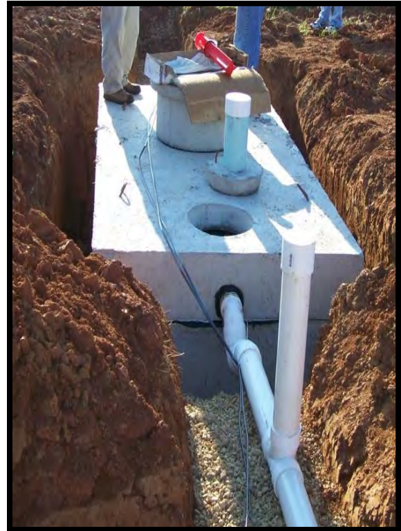
Installation of a 1,000 gallon concrete septic tank.
